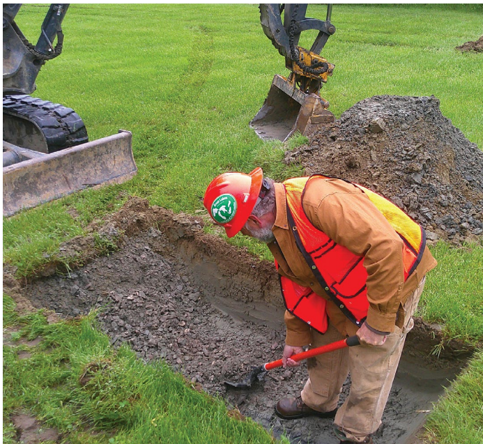
MDB engineer examining test pits in Colchester, VT.
