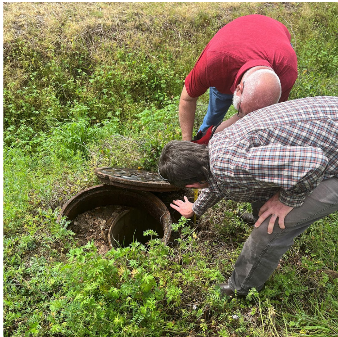
MDB engineer assessing onsite wastewater infrastructure in Duplin County, NC.
